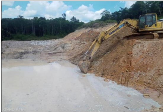
Gambar 6. Pengelolaan Air limpasan Permukaan ( Surface Run Off ) di Area Tambang (Sumber Dept. Environment PT. MME)
